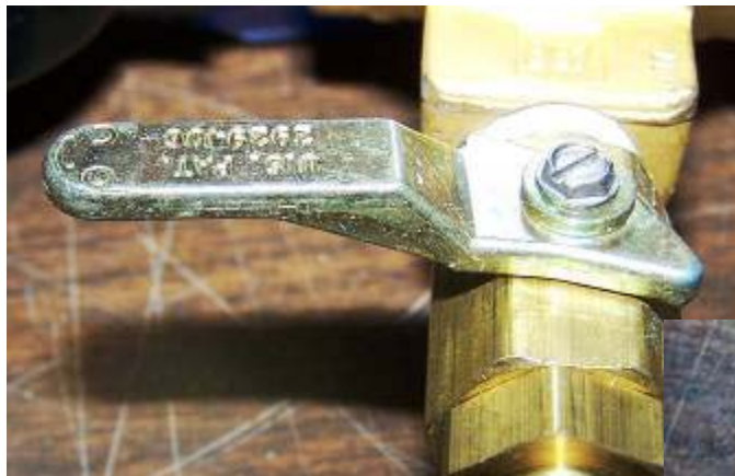
Above: Another type of secondary cut off, again in the "Off" or "Closed" position. You can faintly see an upside down "C" and an "O" at the rounded end of the lever indicating the position.
